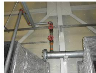
Riser pipe installed from above
