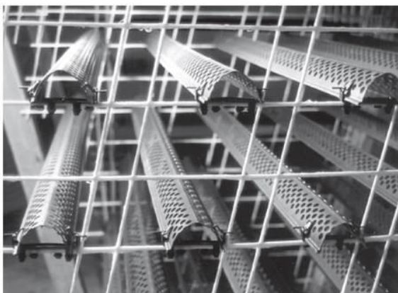
Splash Film Installed
