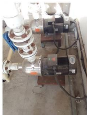
Energy efficient multistage monoblock pump
